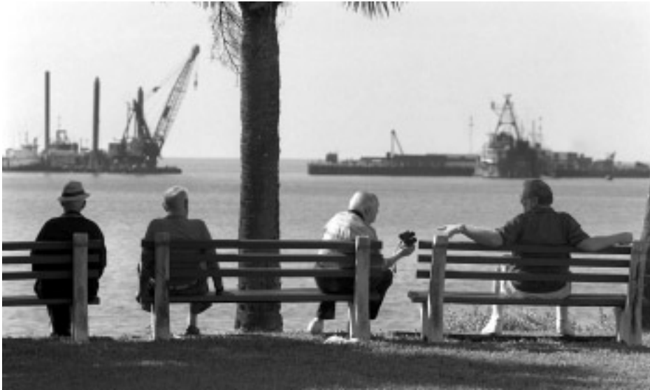
Observers wait for the sand pumping to begin at Golden Beach in Venice. The $28 million project in 1996 moved nearly 2 million cubic yards of sand to widen 3.2 miles of beach.
