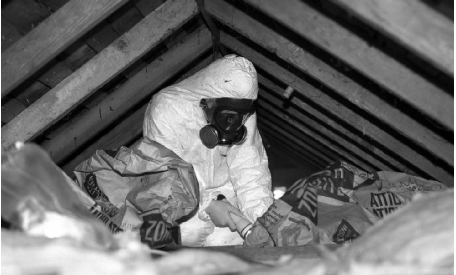
An EPA worker takes samples of Zonolite in a residential attic where the insulation was installed.
