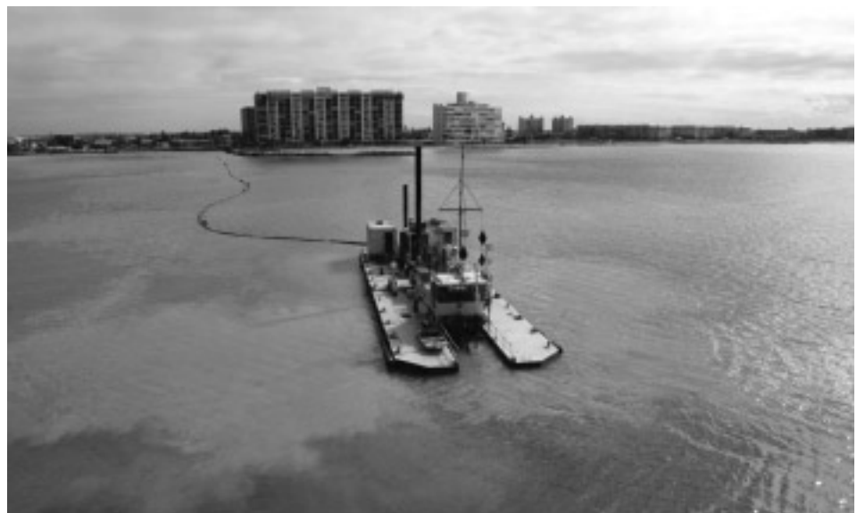
A turbidity cloud surrounds the dredging barge just off shore of the Upton Beach renourishment project in St. Petersburg.
