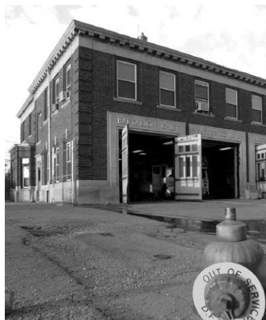
The Detroit Fire Department places the lives of city residents and firefighters in peril everyday because of broken trucks, poor equipment, short staffing and hydrants like this one that do not work.
