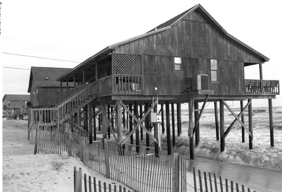
Another barrier island house losing the battle of the tides on Dauphin Island, Ala.
