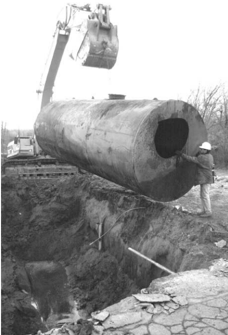
An 8,000-gallon leaking tank is removed from a closed gas station in Independence, Mo.
