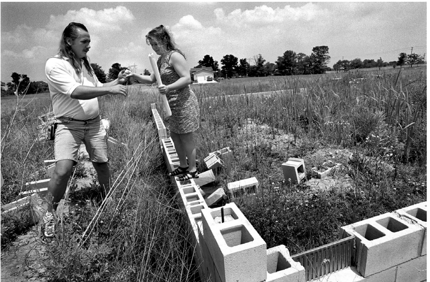
Robert Ratliff helps his wife, Patricia, step over a moat that has developed around a home they were having built. The foundation did not pass inspection, the builders abandoned the project and the Ratliff family was forced to sell the lot. Meanwhile, the attorney general’s office claimed to have saved the couple $288,516.
