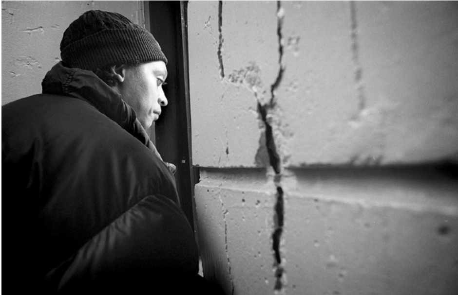
Kenneth H. Parks looks out a window in a cracked dorm building on campus.
