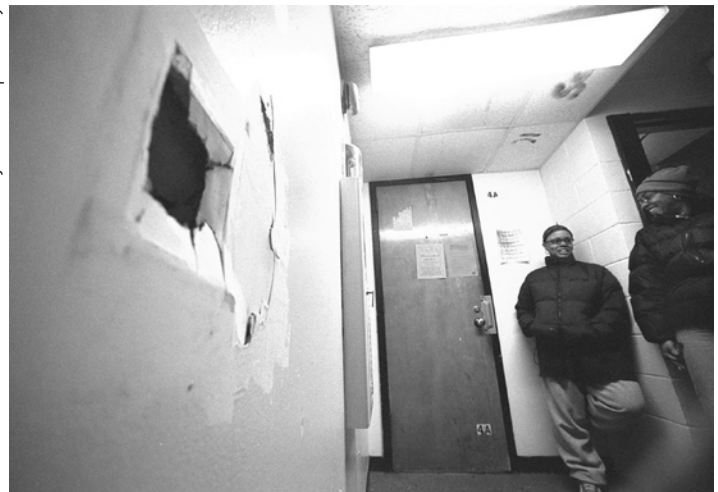
Nadia Reguford (left) and Rochelle Higgs stand outside their dorm entrance where there's a big hole in the wall.
