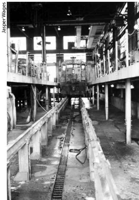
Workers applied chlorinated solvents to locomotives as they were cleaned in railroad shops like this one in Corbin, Ky. The fumes would settle in the pits below.
