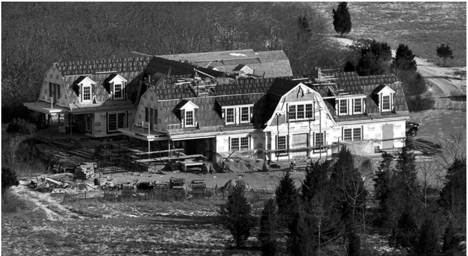
The Herring Creek farm property bought by the Nature Conservancy on Martha's Vineyard, Mass. The house under construction belongs to Daniel W. Stanton of Goldman Sachs.
