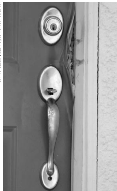
Splintered front door at the site of a home invasion in northwest Las Vegas.
