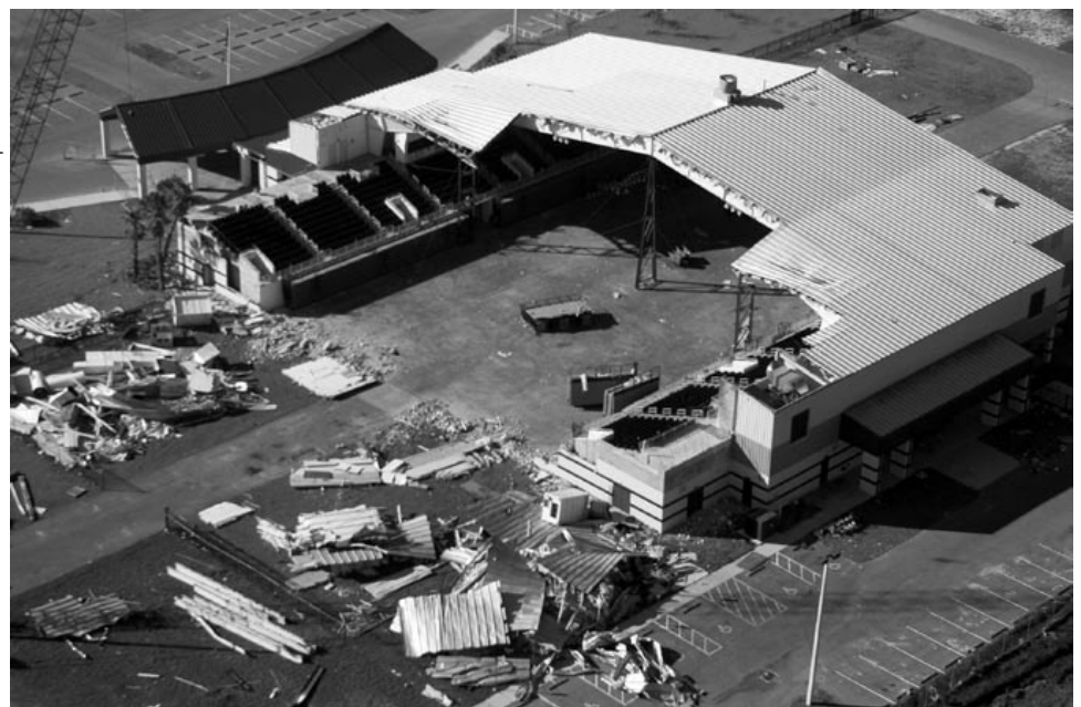
The Turner-Agri Center lies in pieces. It was serving as a hurricane shelter to 1,400 people in Arcadia, Fla., when Hurricane Charley hit with 89-110 mph winds.
