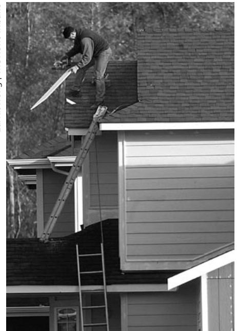
A construction worker – without a safety harness – works atop the second-floor roof of a home being built near Tacoma.
