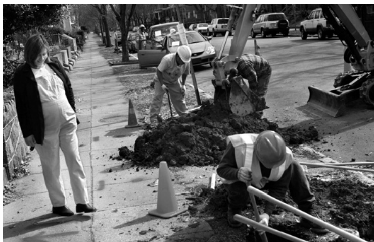
Satu Haase-Webb watches as workers check whether the water pipes to the houses on her block are made of lead. Most of them were. Workers will replace them.
