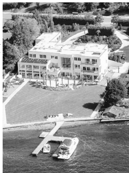
Diamanti, Naveen Jain's 16,500-square-foot mansion on 1.3 acres in Medina, has an indoor pool under a two-story glass atrium, along with a two-story garage, a recording studio and a staff wing.
