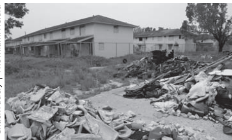
This housing project sits abandoned and covered in trash after it was closed with promises of new housing for its thousands of residents.
