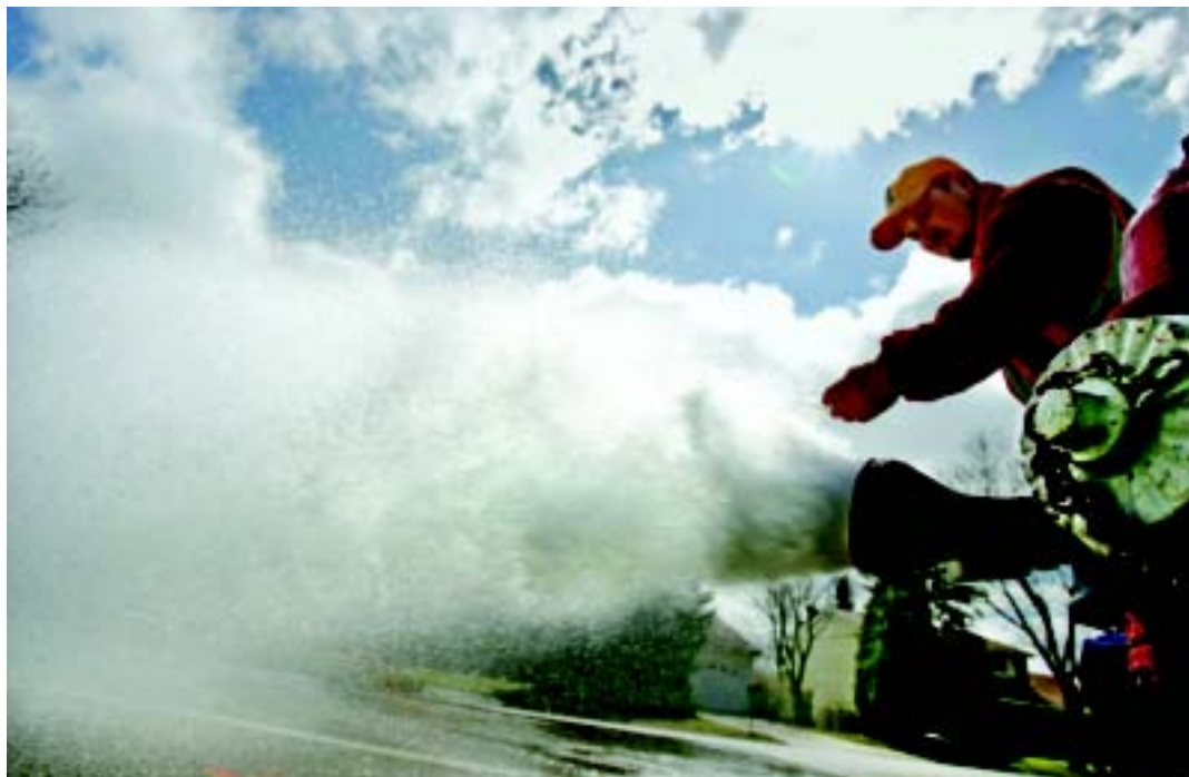
Madison Water Utility employees spent long hours flushing the city's water mains after residents reported manganese in the water supply. A four-part investigative series found additional contaminants, including viruses, in the deep aquifer from which the city draws its drinking water.
