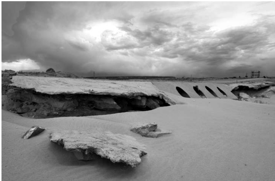
On July 16, 1979, the channel of the Puerco River, which runs along the southern boundary of the Navajo reservation roared with 93 million gallons of radioactive water. The result was the largest accidental release of radiation in American history.
