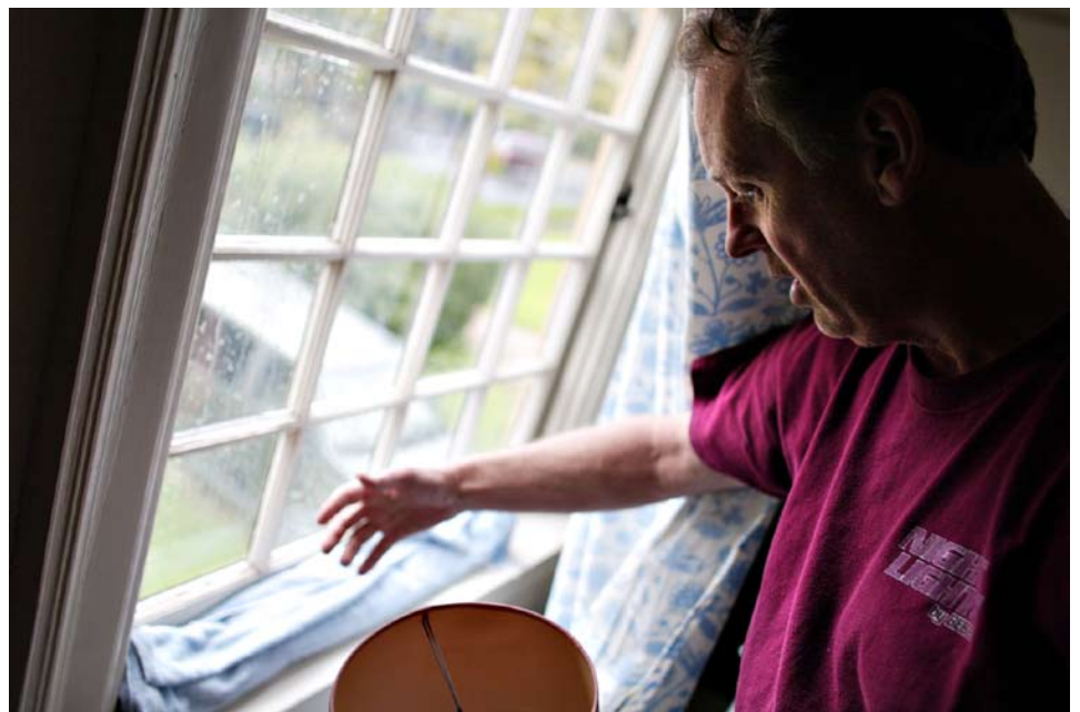
A Caltrans tenant in Pasadena shows the window where he must change towels several times daily to curb the flow of water leaking into his bedroom.
