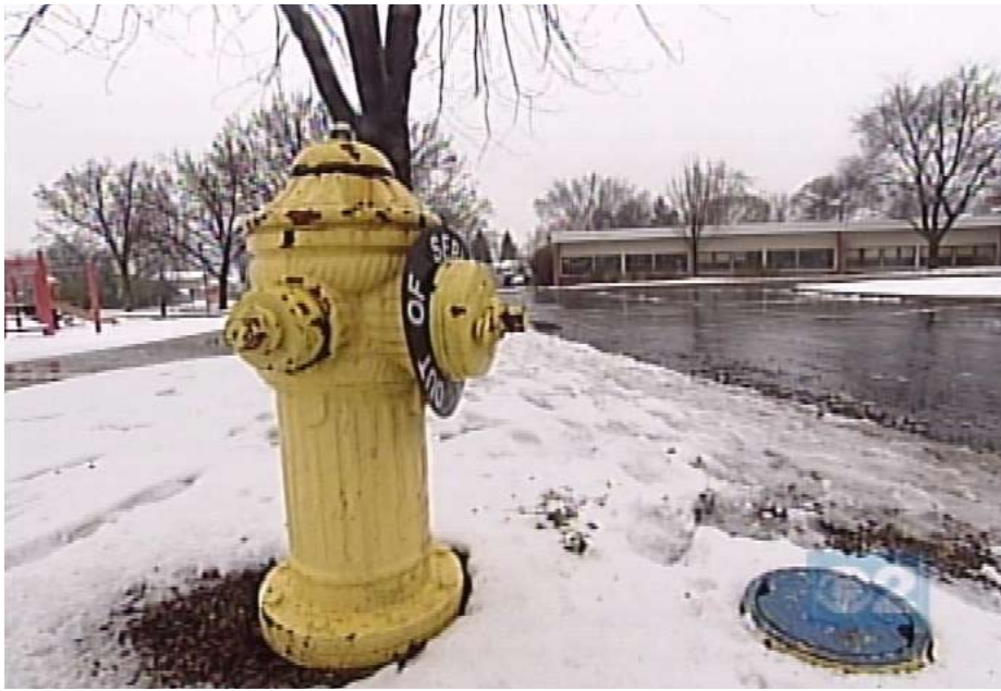
A six-month investigation showed that the Illinois American Water Company failed to inform fire officials about broken hydrants near schools.
