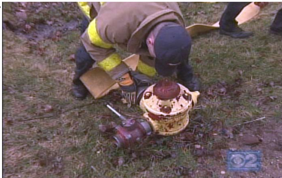
Alerted by reporters, fire departments flagged broken hydrants, but they have no authority over the private companies responsible for repairs.
