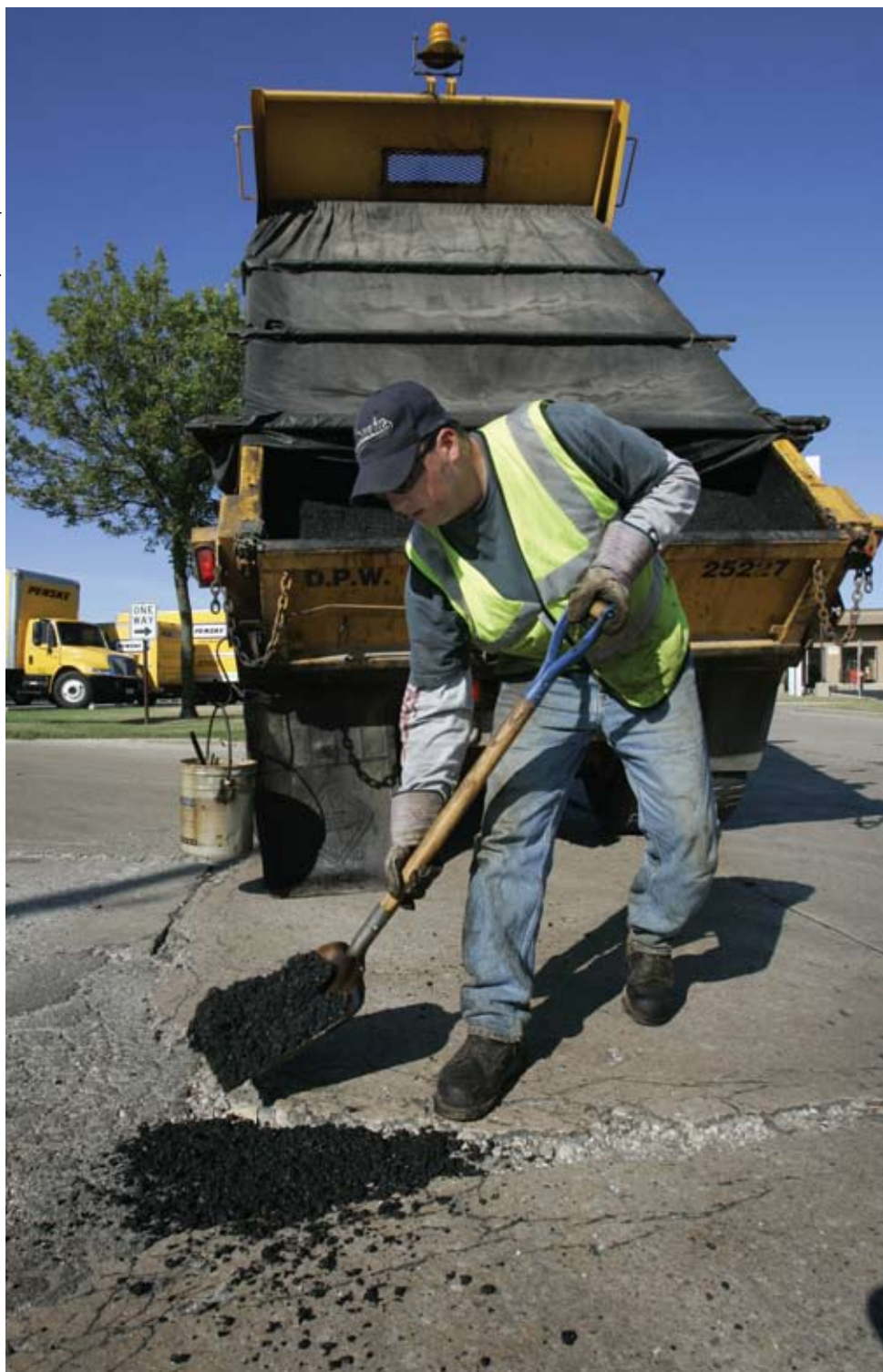
Craig Maier, a worker with the City of Milwaukee, fills potholes on a stretch of W. Carmen Avenue.
