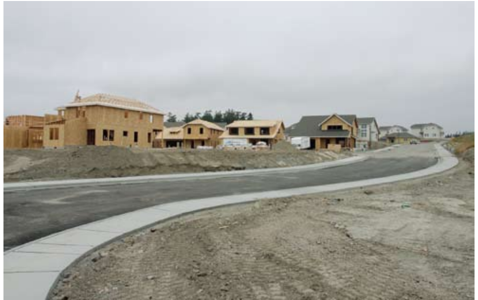
Homes are under construction in the Crescent Harbor area at Naval Air Station Whidbey in Oak Harbor. Contractor Forest City is speeding up the work after taking over from the previous builder, American Eagle.
