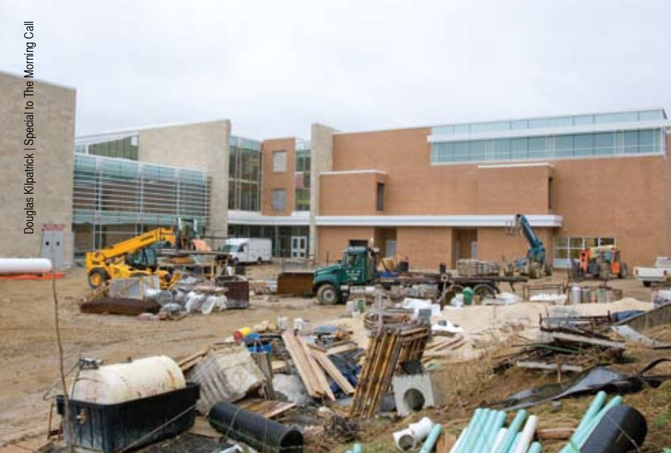
Construction earlier this year of a new $55 million Broughal Middle School in Bethlehem, Pa.
