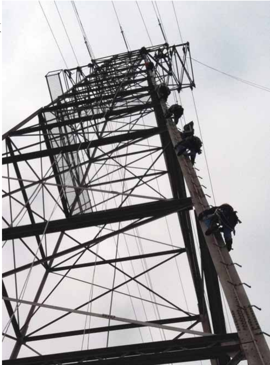
Seattle City Light lineworkers head to work 180 feet off the ground. They don't clip in their safety harnesses until they finish the eight-minute climb.
