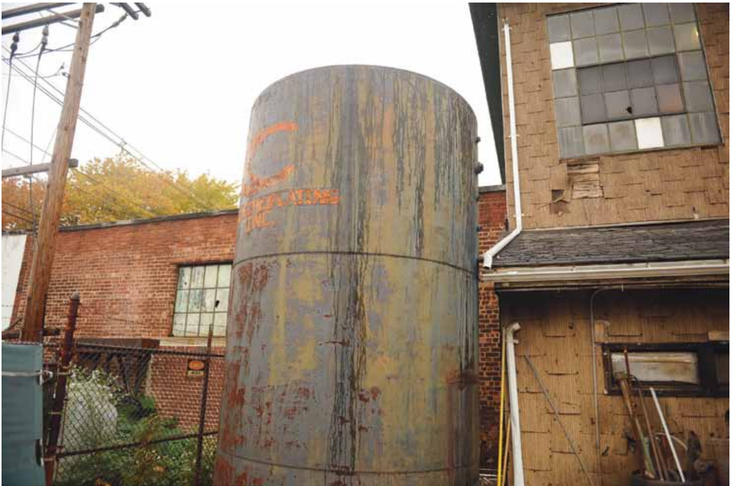
This tank was the source of the 1983 leak, according to the EPA. The site was named a Superfund site in September 2011.
