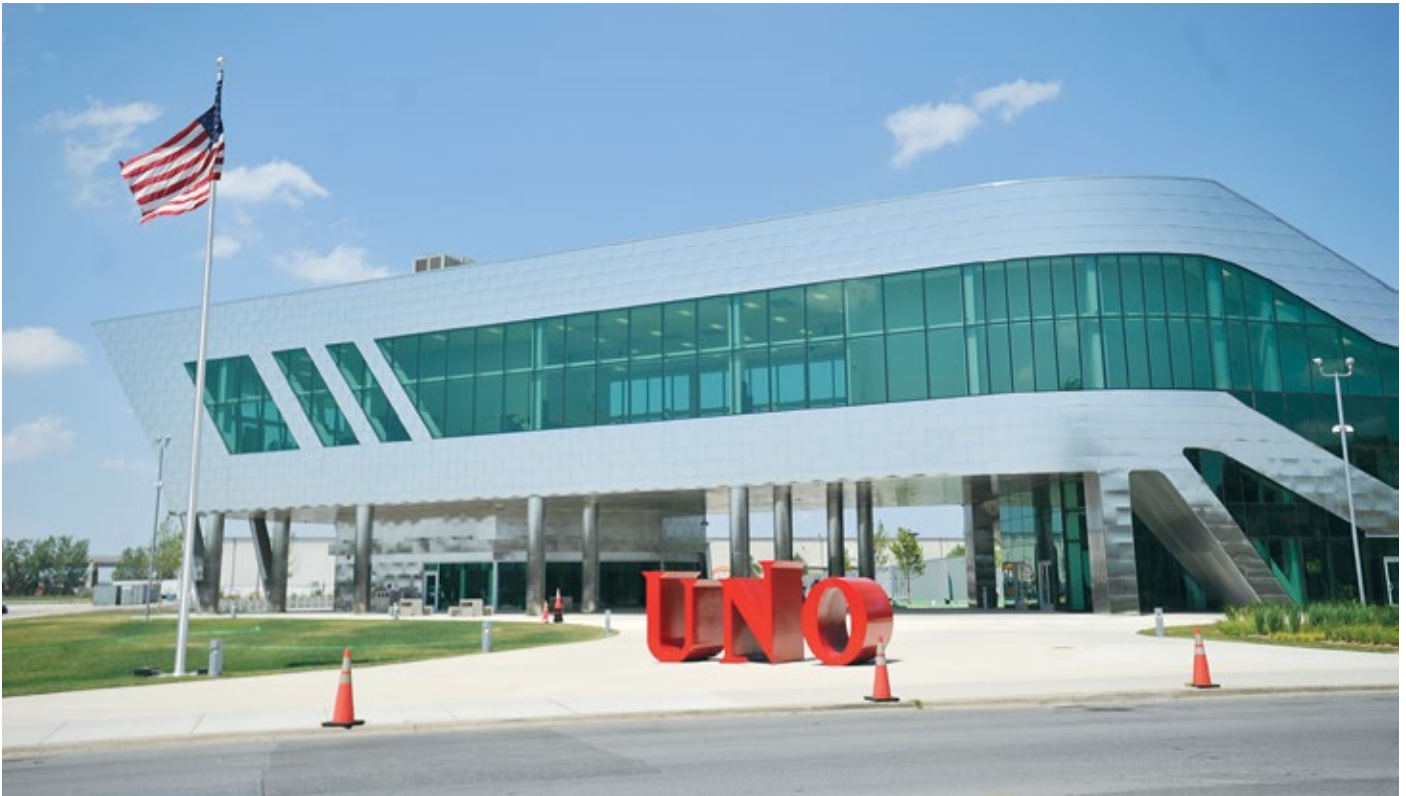
The UNO Soccer Academy was one of the charter schools built with a state school-construction grant that has been heavily scrutinized.
